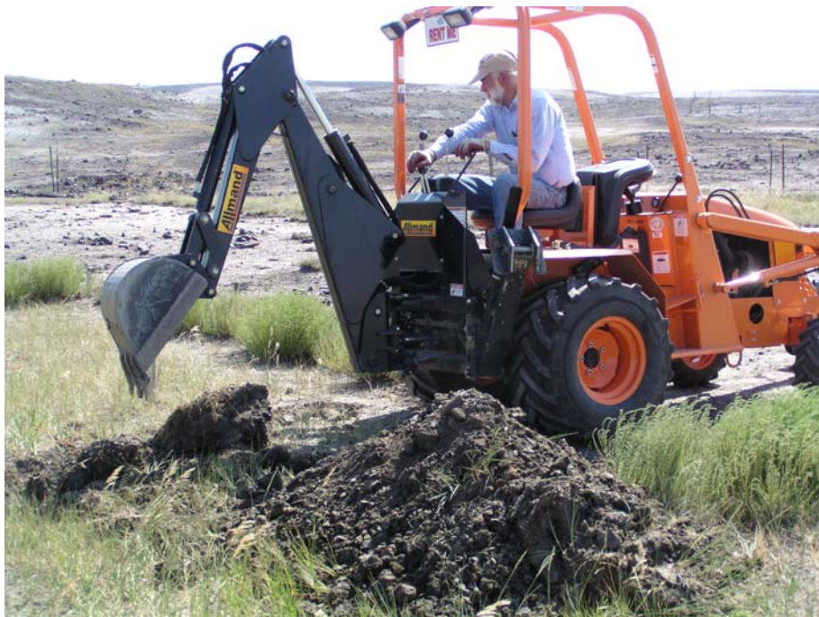
Image 5. Excavation in replication plot 2 of Treatment 7 in preparation for soil sampling and root evaluations.
