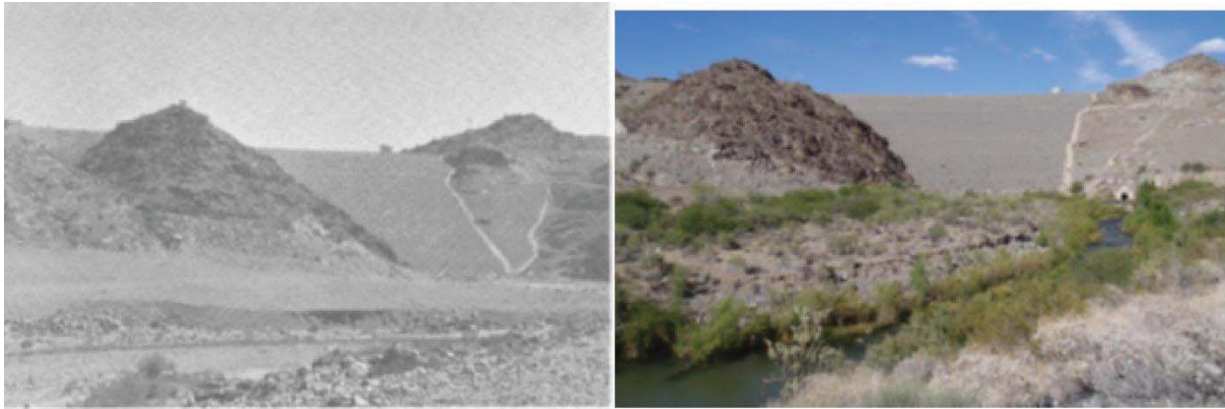
46. Alamo Dam; downstream side.
