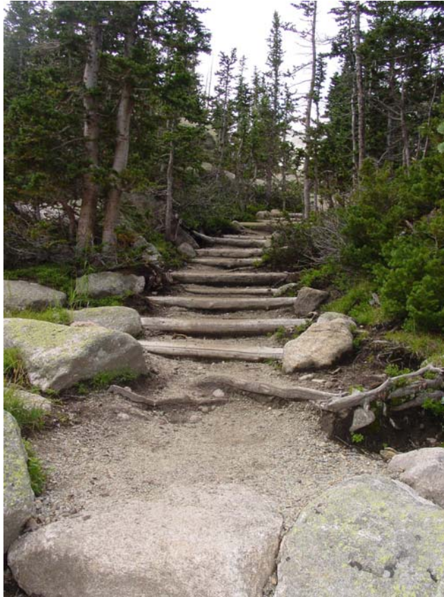
Figure 51. Example of retainer bars constructed below the natural grade
