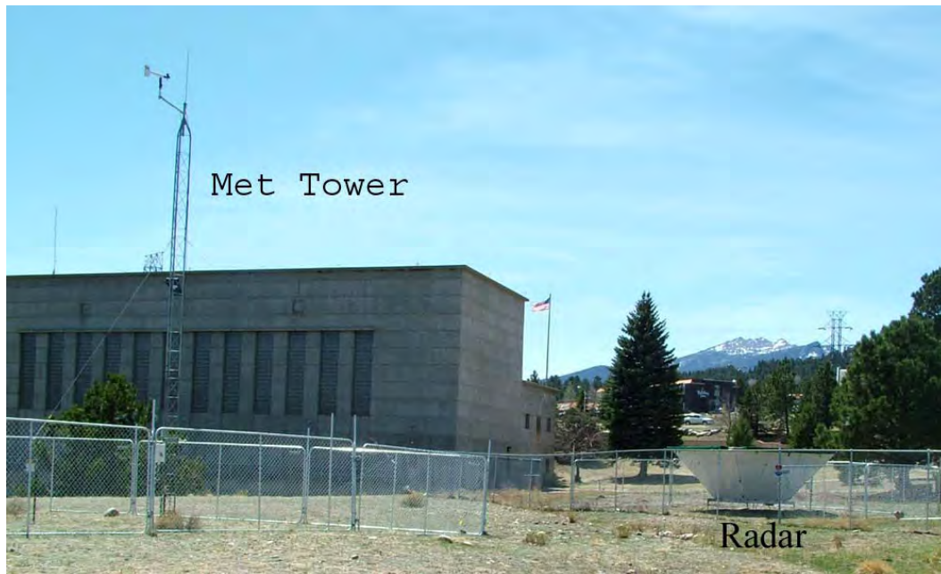
Figure 2.4. Radar wind profiler and 10-m meteorological tower in Estes Park, Colorado.
