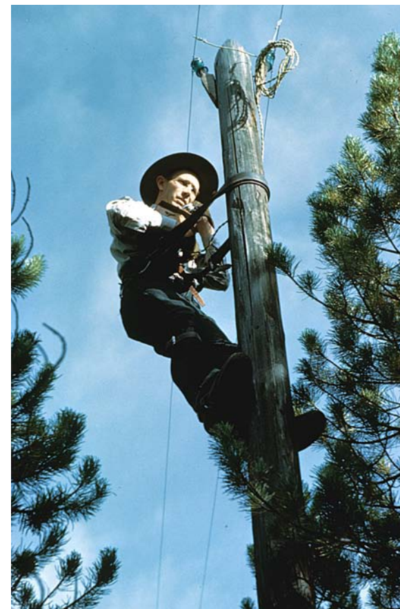
Lineman engaged in telephone repair, 1946. The park continued to maintain a phone line to the Boulderfield throughout the 1930s and 1940s, though adverse weather conditions meant that the line needed frequent repair. This photo may not have been taken on Longs Peak, but it provides an image of a type of maintenance work that was commonplace in the park’s backcountry at mid-century. Image courtesy of Rocky Mountain National Park.
