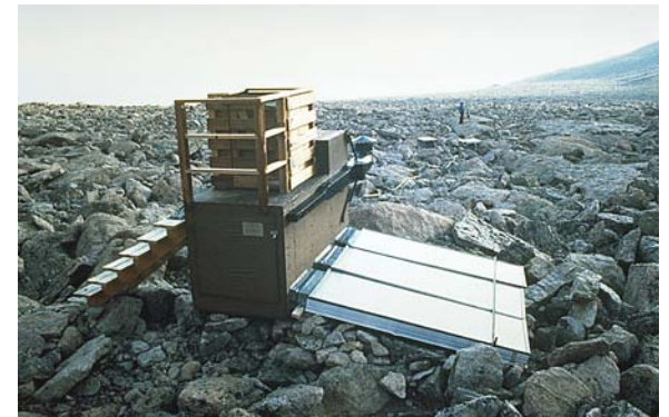
Solar toilet at the Boulderfield, Longs Peak, 1985. Park rangers replaced the vault toilets at Chasm Junction and the Boulderfield with dehydrating solar toilets in the mid 1980s, hoping to reduce the impact of human waste on the backcountry. Image courtesy of Rocky Mountain National Park.
