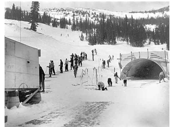
Hidden Valley Ski Area, Tunnel and Upper Slopes, 1954. Hidden Valley was not formally part of Mission 66, but it reflected a similar commitment to developing recreational facilities in frontcountry portions of the park. Image courtesy of Rocky Mountain National Park.
