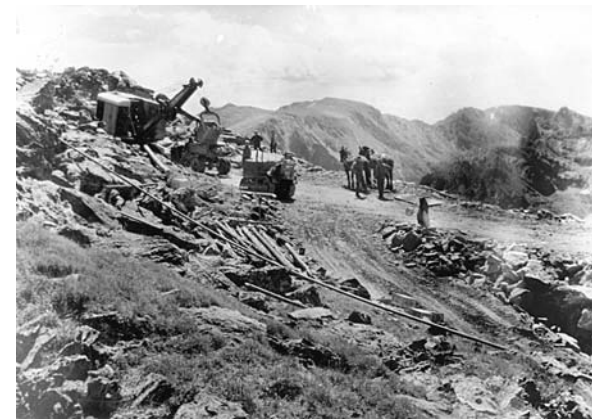
Construction of Trail Ridge Road, 1930s. The construction of Trail Ridge Road was the most important development in Rocky Mountain National Park in the 1930s. The road signaled the park’s growing commitment to serving automobile tourists. The road quickly became the new centerpiece of the park, lessening the significance of Longs Peak. Image courtesy of Rocky Mountain National Park.
