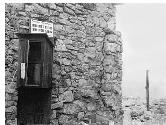
Boulderfield Shelter Cabin, showing evidence of structural damage, 1936. The Boulderfield cabin, though popular with climbers and often filled beyond capacity, was quickly breaking apart because of the shifting glacial field on which it was built. The cabin was taken out of service and dismantled by the end of the 1936 summer climbing season. Image courtesy of Rocky Mountain National Park.
