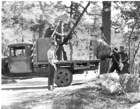
Emergency Conservation Workers Loading Boulder Truck, 1936. Like CCC workers, EC workers devoted a great deal of time to the construction and improvement of roads and bridges in Rocky Mountain National Park. Image courtesy of Rocky Mountain National Park.
