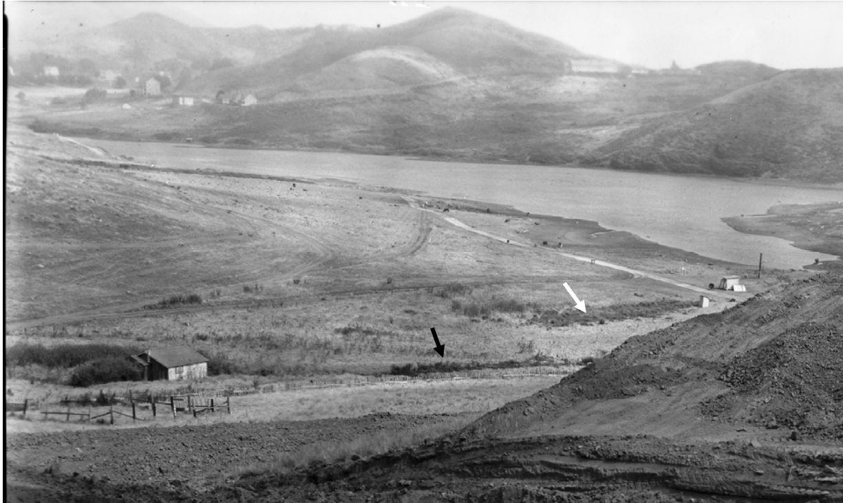
Figure 4. August 31, 1938. Looking southeast to the area down valley (south) of the ranch road (out of frame left). Arrows highlight drainage features visible in Figures 2 and 3. Black arrow shows a ditch below the small building. White arrow points to a natural historic drainage.
