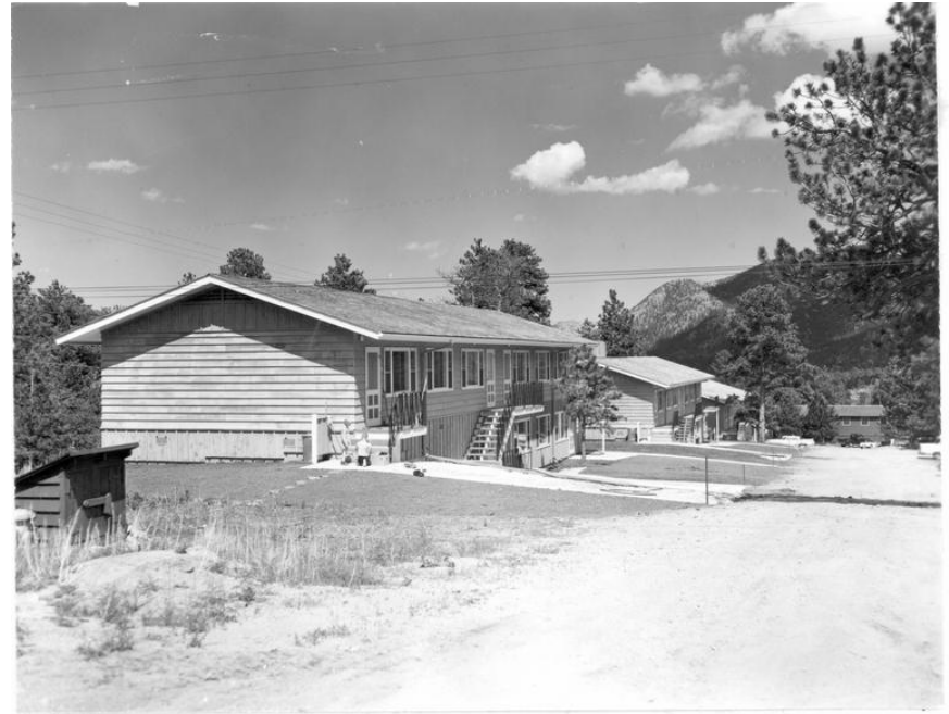
Multiple-unit residential buildings constructed on Sundance Circle, 1963 Photo courtesy of Rocky Mountain National Park
