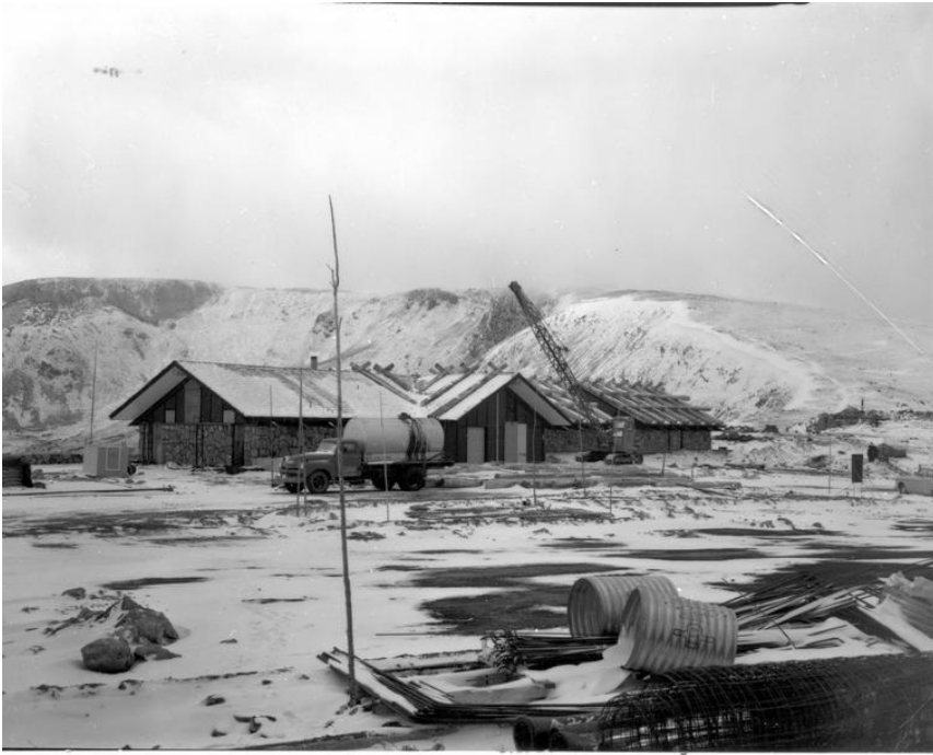
Construction of the Alpine Visitor Center at Fall River Pass, 1963 Photo courtesy Rocky Mountain National Park
