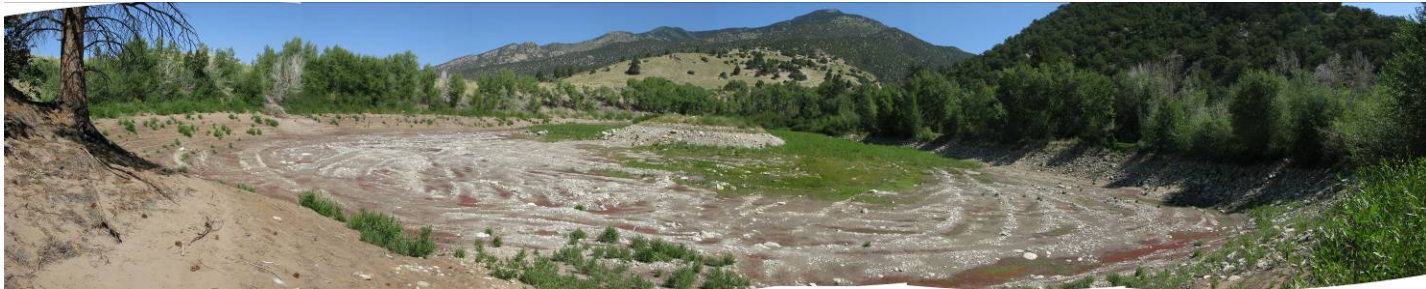
Pit 7 (above) looking east. Levee is on right below trees, dike is the vantage point from which photo is taken, and island can be seen as gravel area within green vegetation. Sand Creek is to right of levee.
