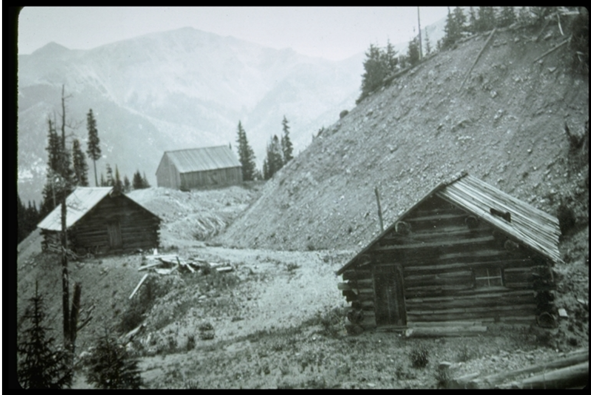
This undated photograph documents several important features of the Grand Ditch. Note the large right-of-way, the steep slopes of ground denuded of timber, the rough character of the banks of the ditch itself, and the log cabins used by the workers who inhabited this ditch camp. Photographer unknown, n.d., catalog #10-D-606, RMNP Photo Collection.
