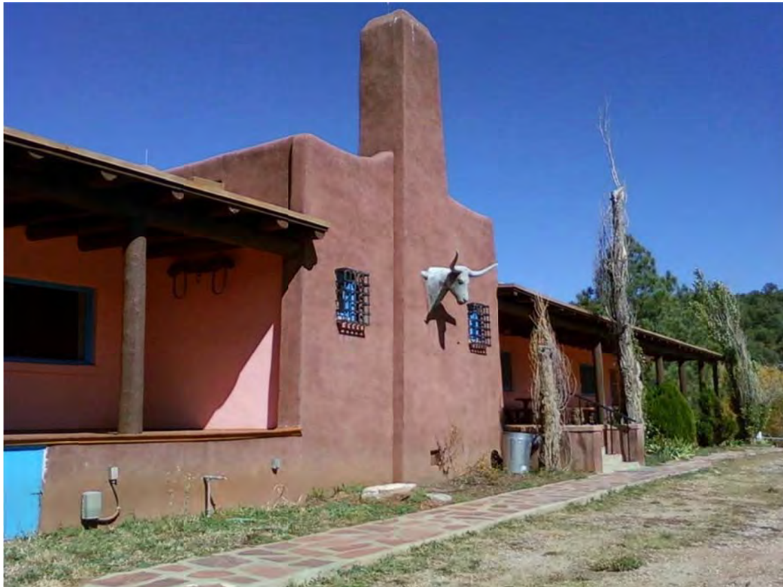
Exterior of the Forked Lightning Ranch House. Photo by Maren Bzdek.
