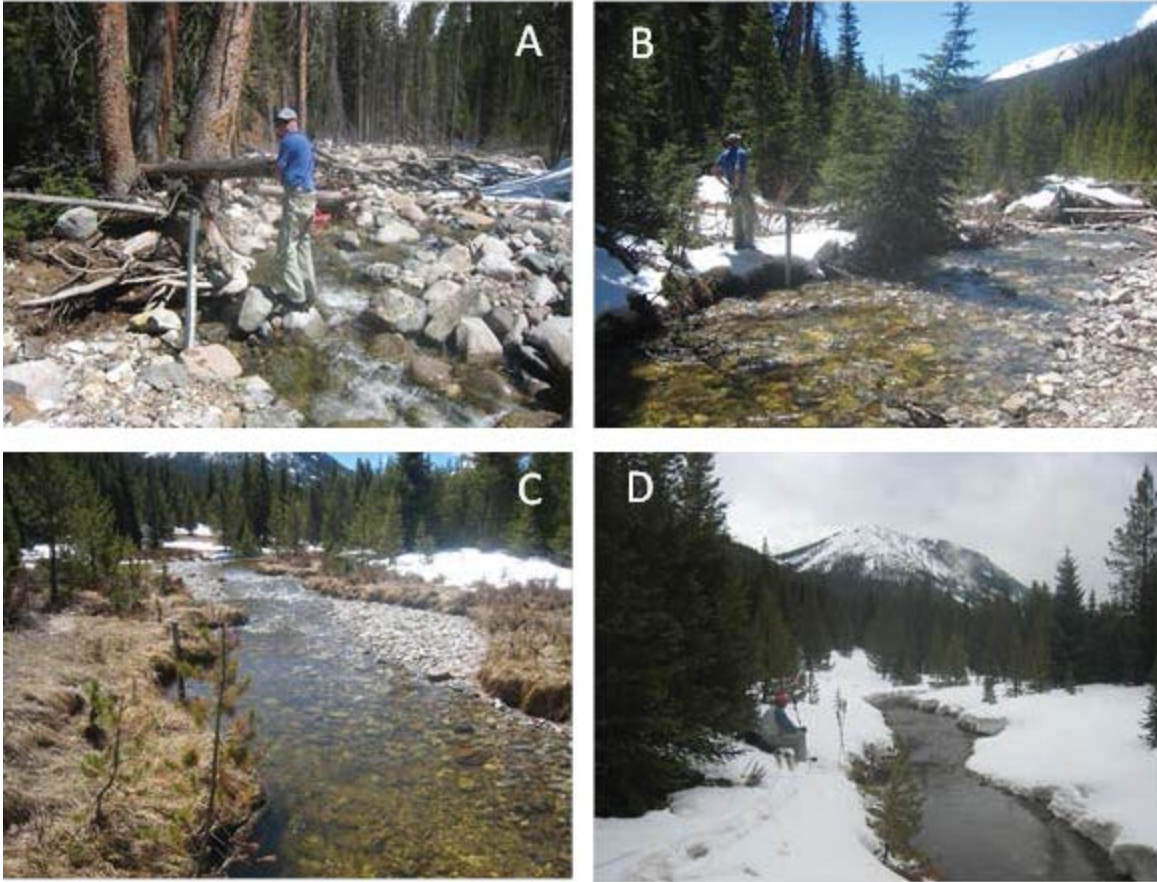
Figure 2. New gauge installation on April 22, 2012 at A) Lower Lulu, B) Crooked Tree, and C) Gravel Beach (gauge is on left bank behind small tree). In image D) taken on May 7, 2013, a pressure transducer was placed in the Gravel Beach gauge prior to snowmelt. View in all images is downstream.
