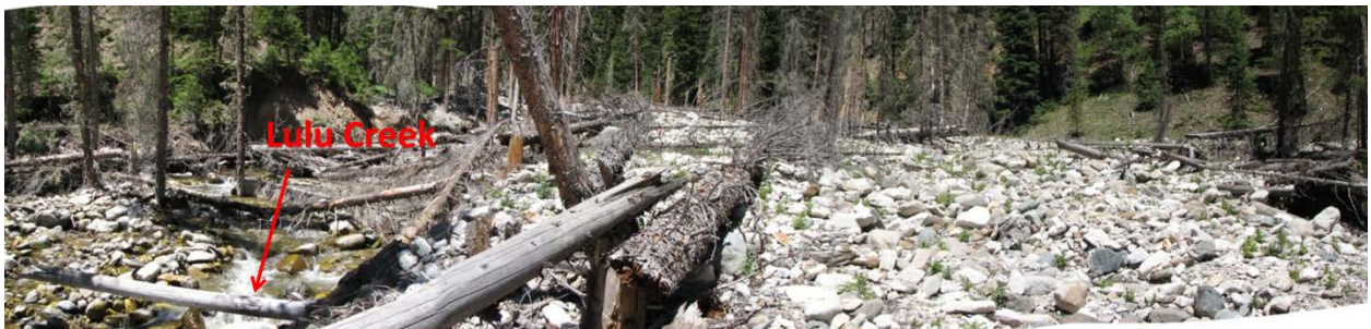
Figure 6. Upstream view of Lulu Creek showing the existing condition of the left overbank area.
