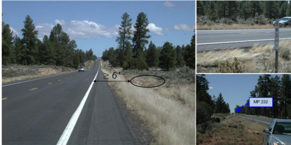
Figure 7: DMS Location on Site 3
