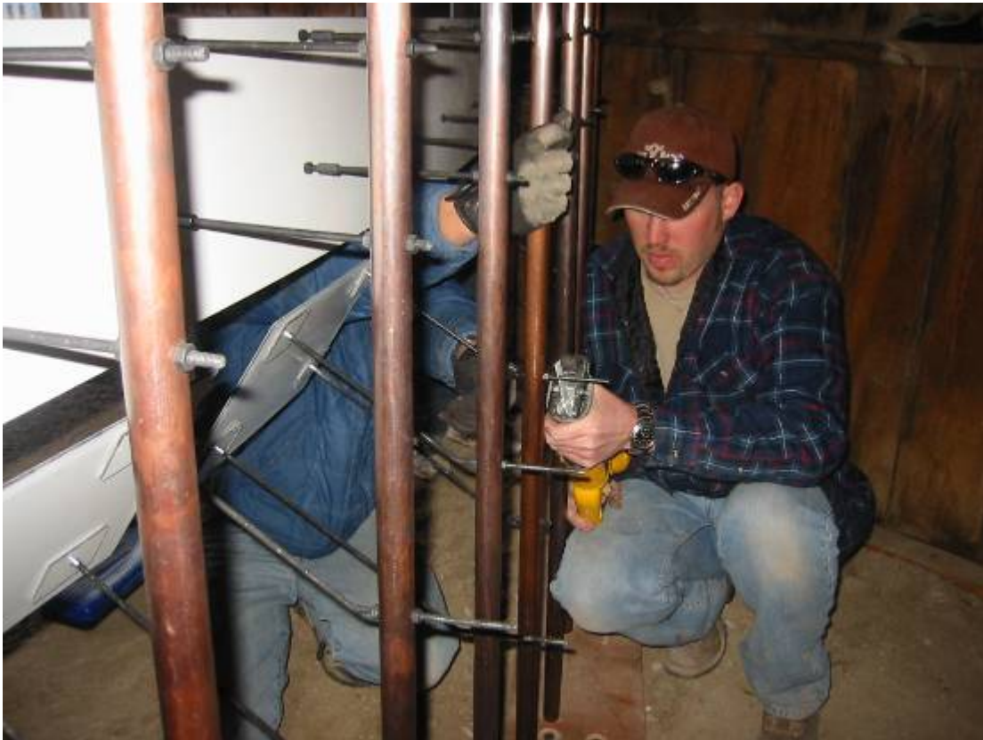
Trimming all-thread connections to address safety concerns.
