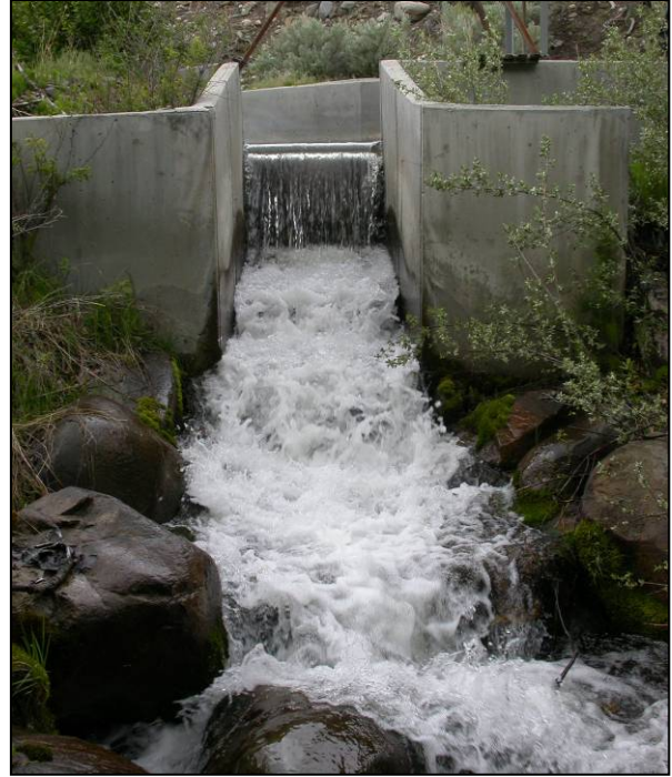
Image 12. The third irrigation diversion on Reese Creek. Species composition above and below the diversion indicate that it is a barrier to upstream fish movement, but electrophoretic genetic results reveal hybridization has occurred above the diversion.
