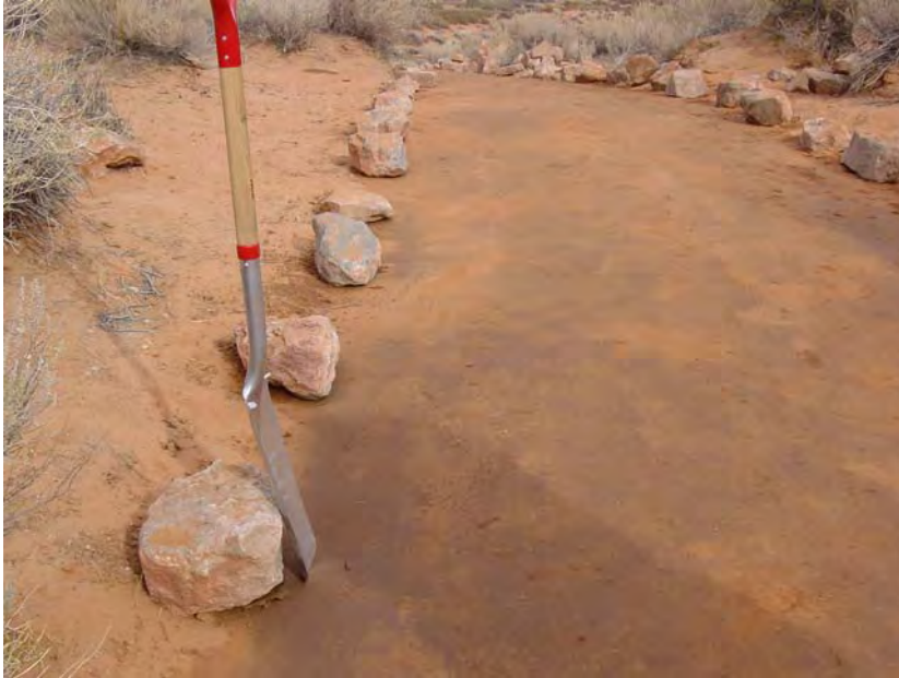
Chemical trail stabilization including rock borders.
