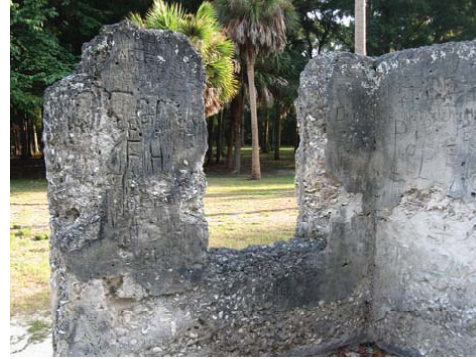
Evidence of vandalism in a slave cabin
