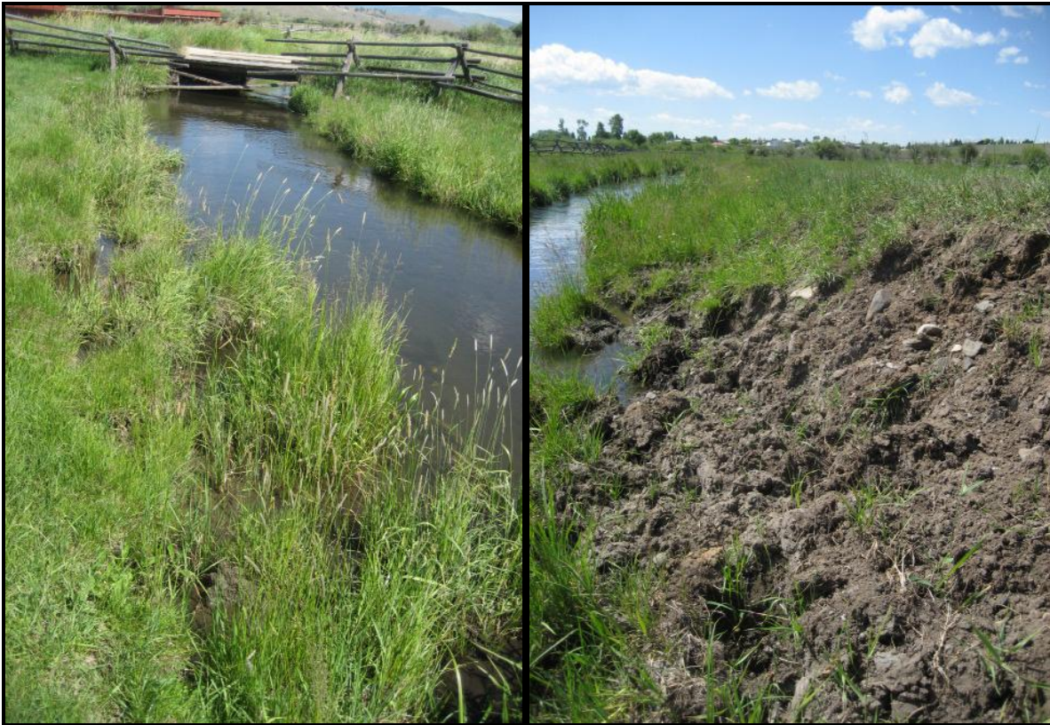
Photo 2. Pugging and hummocking along the Kohrs-Manning Ditch in the Stuart Annex Field at the Clark Fork River Bridge Road.
