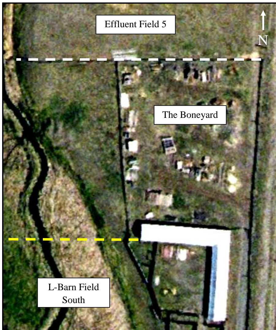
Photo 6. Historical and current southern boundaries (yellow and white lines, respectively) of Effluent Field 5.
