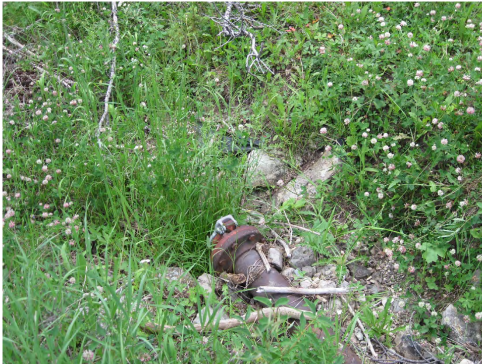
Figure 6. Water pipe in treated area
