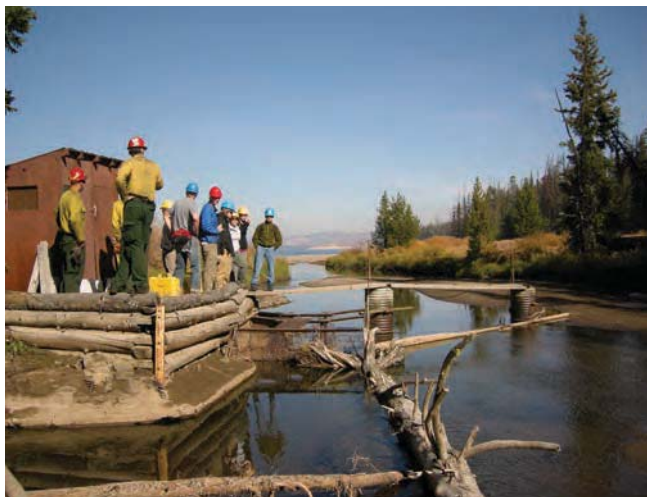
Students from Montana State University's Department of Civil Engineering assess damaged supporting structures at the Clear Creek weir site, while firefighters (left) look on.
