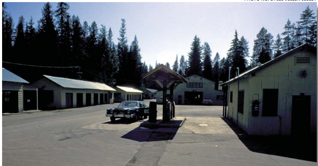
Figure 26. View west of the older utility yard, 1983.
