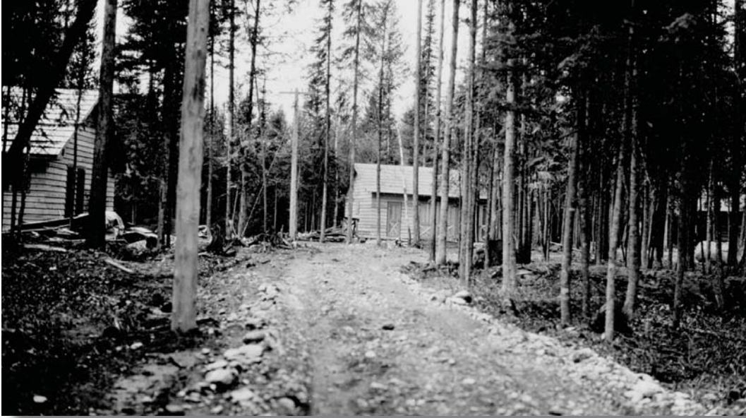
Figure 2. The headquarters site featured level ground and a “dog-hair” growth of lodgepole pine, as seen in this 1929 construction photo. The road is probably today’s Ruhle Drive.
