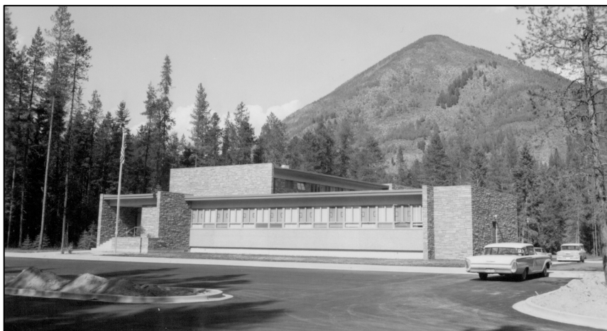
Figure 22. Administration building, front and side views. Photo taken by John Palmer, August 1963. Photo No. 8493.
