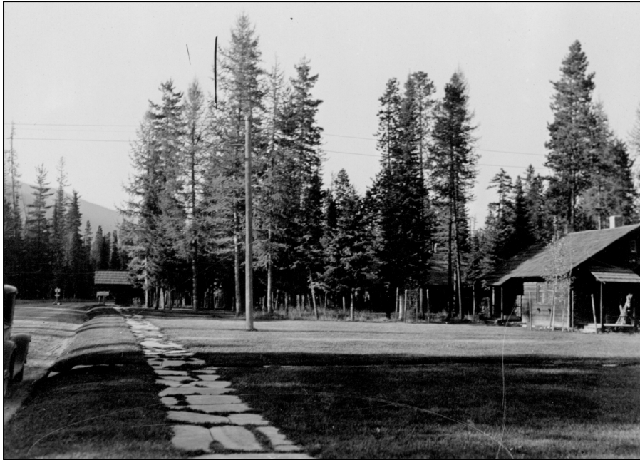
Figure 12. Flagstone path. View north Mather Drive, September 1934. Photo caption states that it was built by CCC camp NP 1. Photo No. HPF 2185.
