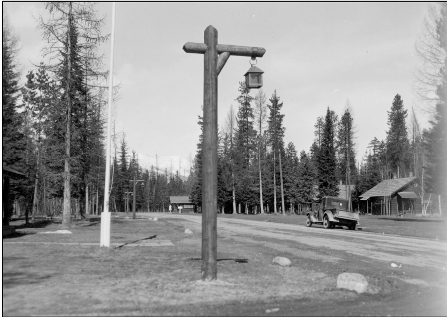
Figure 13. Street lights. View north along Mather Drive. Photo No. HPF 1904.
