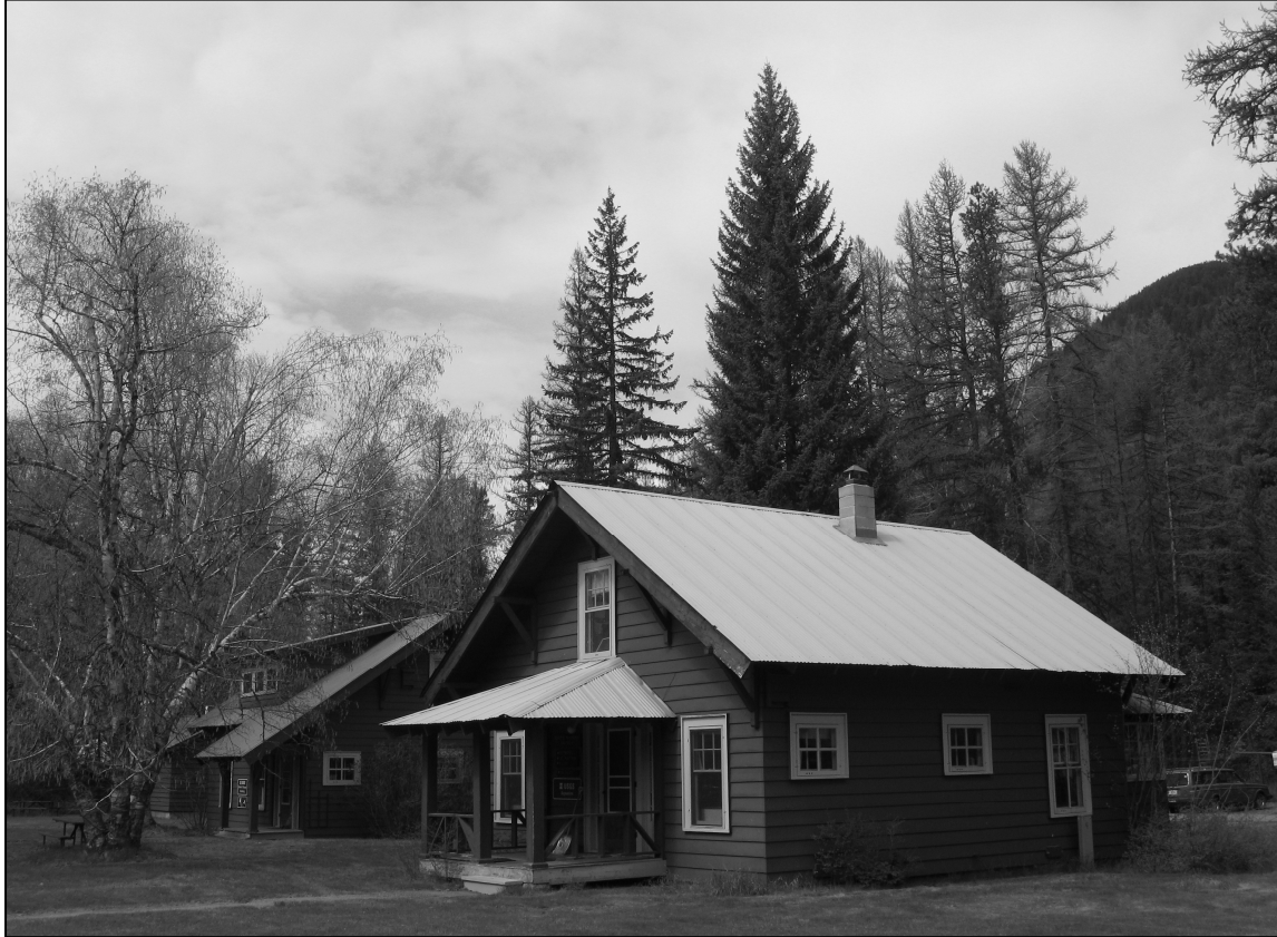
Figure 4. View north of two offices and former ranger residences (Buildings 3 and 4) showing the forest and mountain-view setting. Photo taken on centennial anniversary, May 10, 2010. Photo by Ted Catton.
