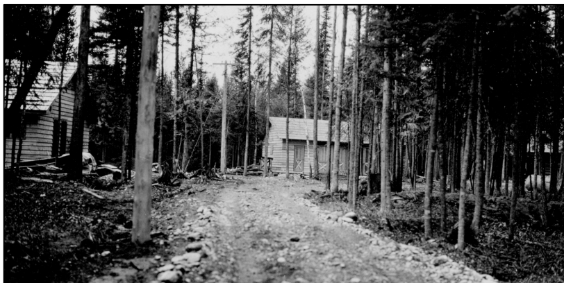
Figure 3. The site featured level ground and a “dog hair” growth of lodgepole pine as seen in this 1929 construction photo. The road is probably today’s Ruhle Drive. Photo No. GLAC 15502-C.
