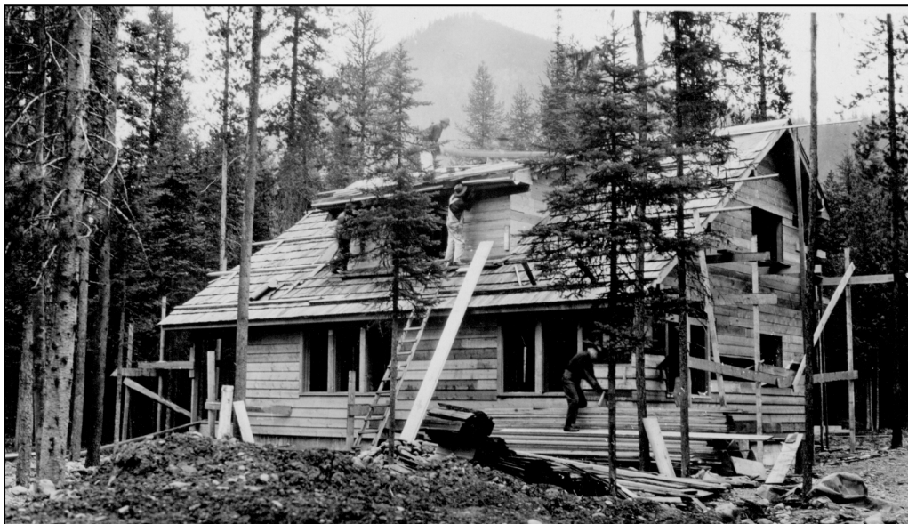
Figure 2. U.S. Commissioner’s residence (Building 9) under construction in 1929. Trees were preserved during site development, and eighty years later the cultural landscape is still dominated by the deep forest setting. Photo No. GLAC 15502-B.
