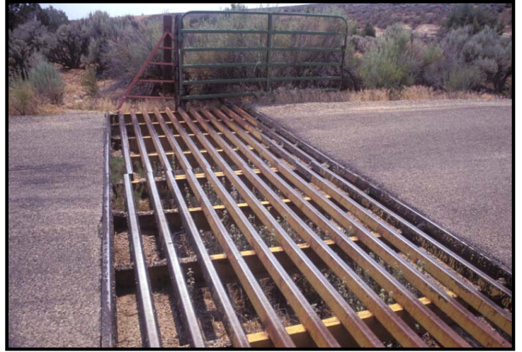
Figure 6. Marrubium vulgare growing underneath cattle guard at entrance to the Square Tower Group and visitor center. (HOVE PR-4)
