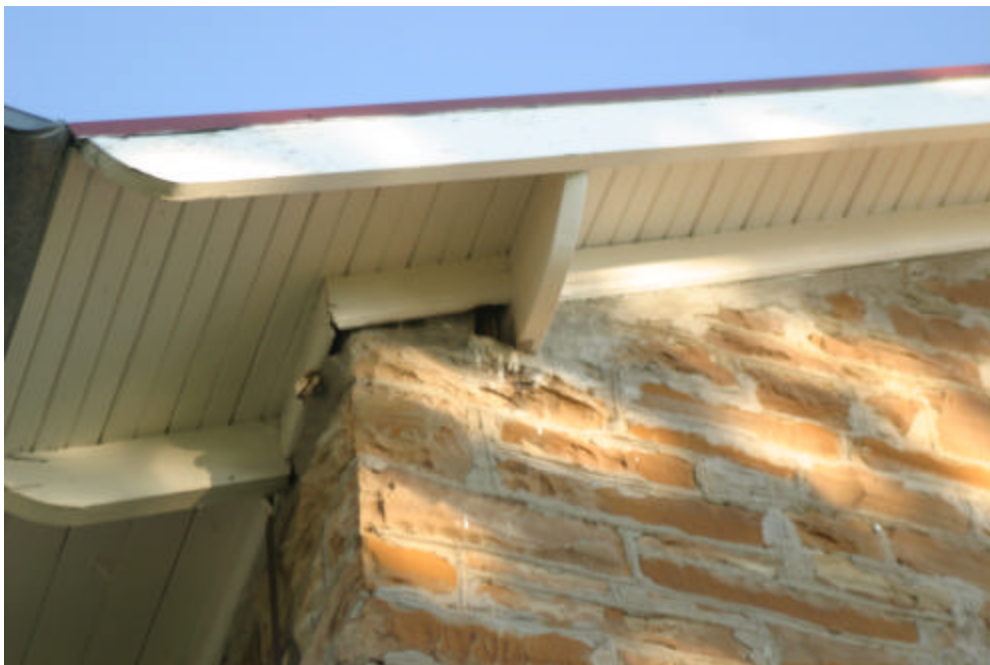
Fig. 6. Eaves of White Swan Library, showing bat guano and entry points used by roosting big brown bats.
