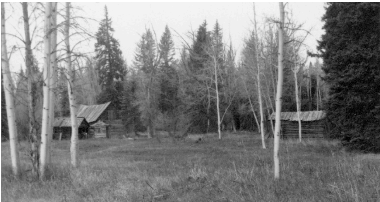
View of western portion of Murie Ranch Historic District. Only the Frame Cabin, #991 (far left of cluster) survives. The adjacent Barn, #990 and Storage Shed, #989 (barely visible between barn and Frame Cabin), were removed in the late 1970s, and the non-contributing Oil House, #988 (far right) has been burned since 1998. (Photo taken 1977; GRTE archives)
