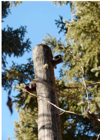
Early electric pole: left image shows the top, with ceramic insulator, and right shows base supported by extra post.
