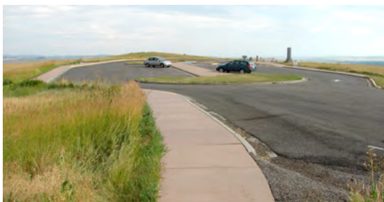
Asphalt parking lot and concrete sidewalks on the Reno-Benteen site exhibit materials and scale outside the period of significance.
