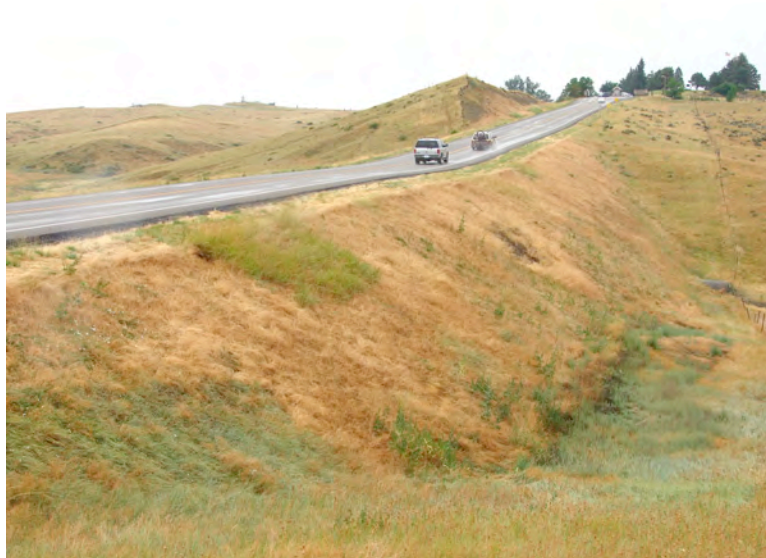
Cut and fill along LIBI entry road
