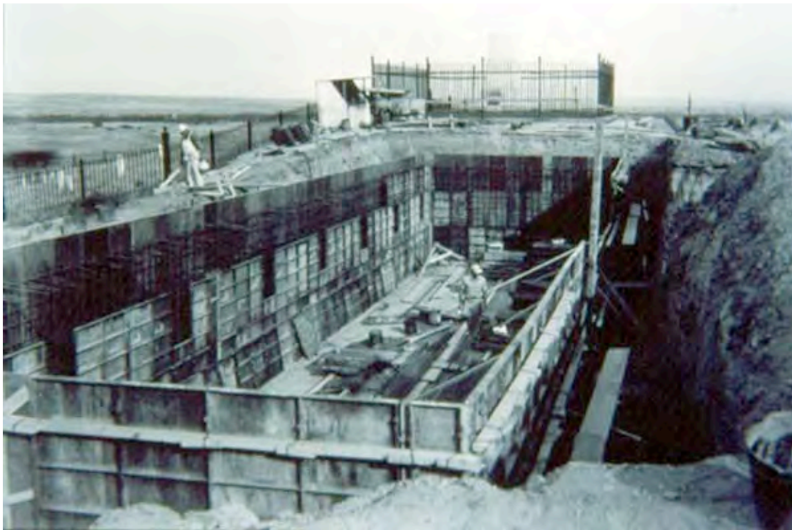
Underground water reservoir on top of Last Stand Hill under construction in 1952/53. Note proximity to battlefield on left and Custer Monument above. Source: LIBI archives
