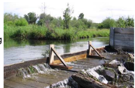
The Kohrs-Manning Ditch, which originates on the park and carries water to four ranches, pulls water from the Clark Fork River
