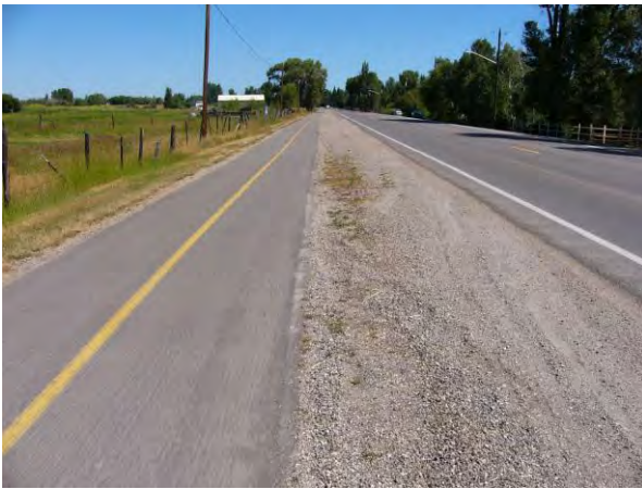
Typical constructed pathway near Garden City.
