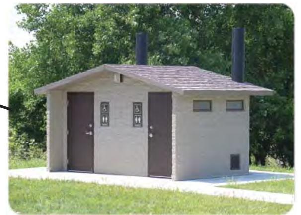
Vault Toilet - CXT Tioga w/chase funded through UT State Parks
