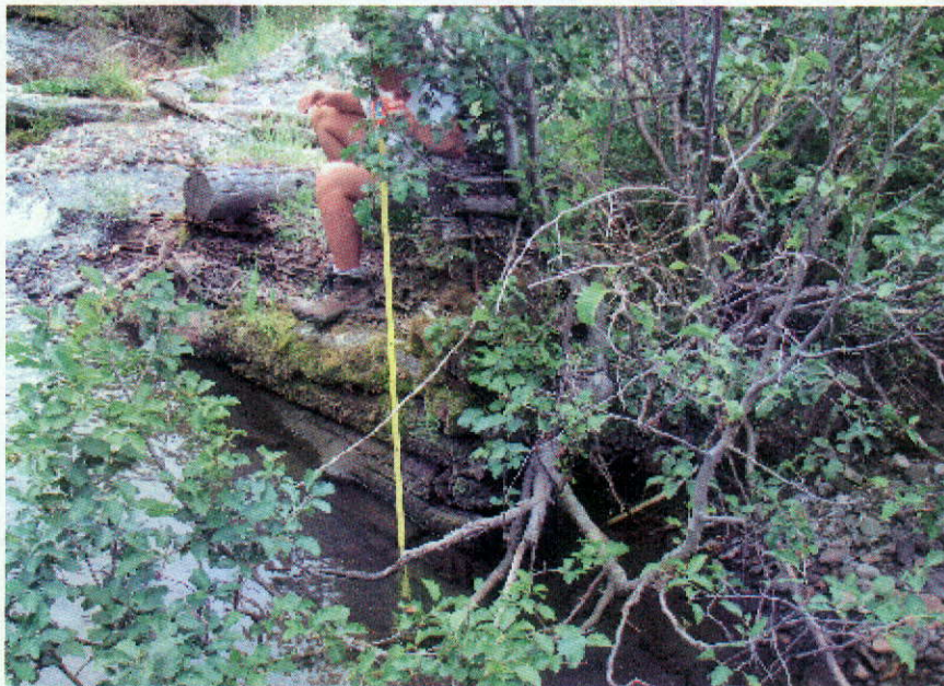
West corner bridge abutment.
