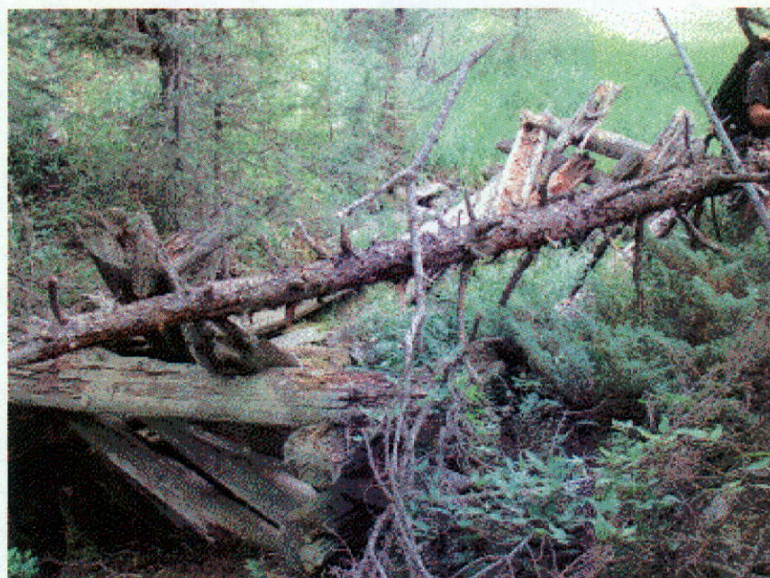
Crib log pier side wall view.
