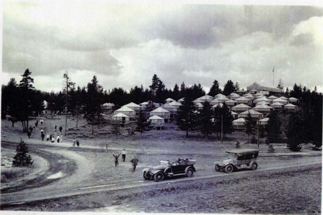
View to the northwest at the Wylie Camp on slopes of Wylie Hill in 1915, historic photograph (YELL 50774). Note large dance hall tent on top of hill where Feature 21 lies.
