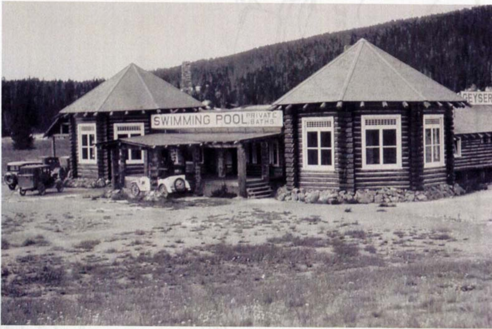
View of the front of the first bathhouse
