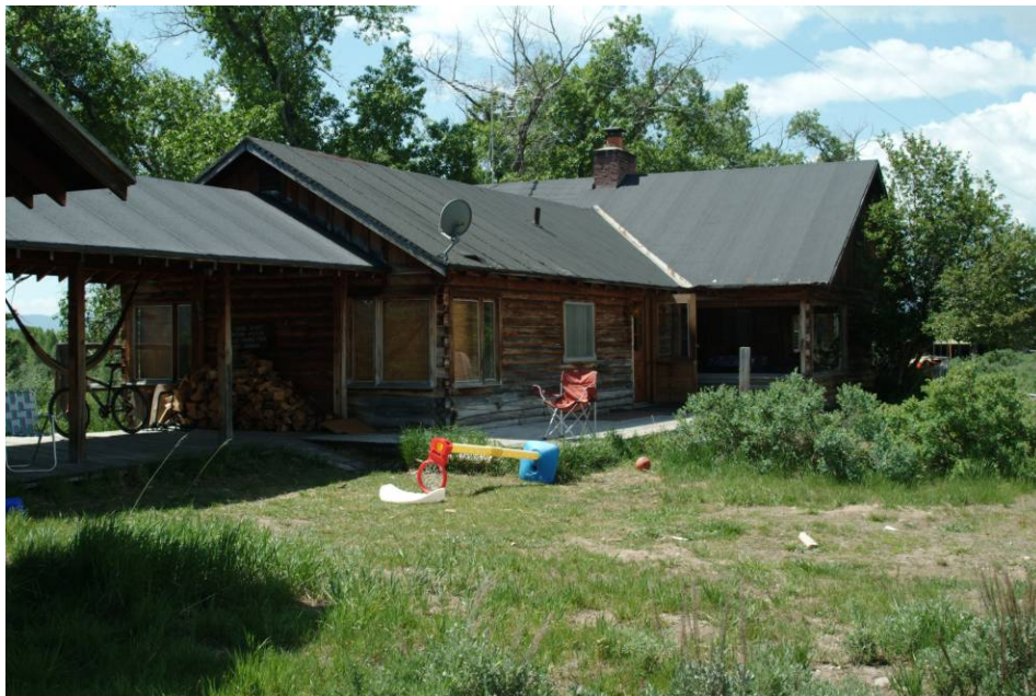
Wittmer House, north and west elevations (Mary Humstone, 2007)
