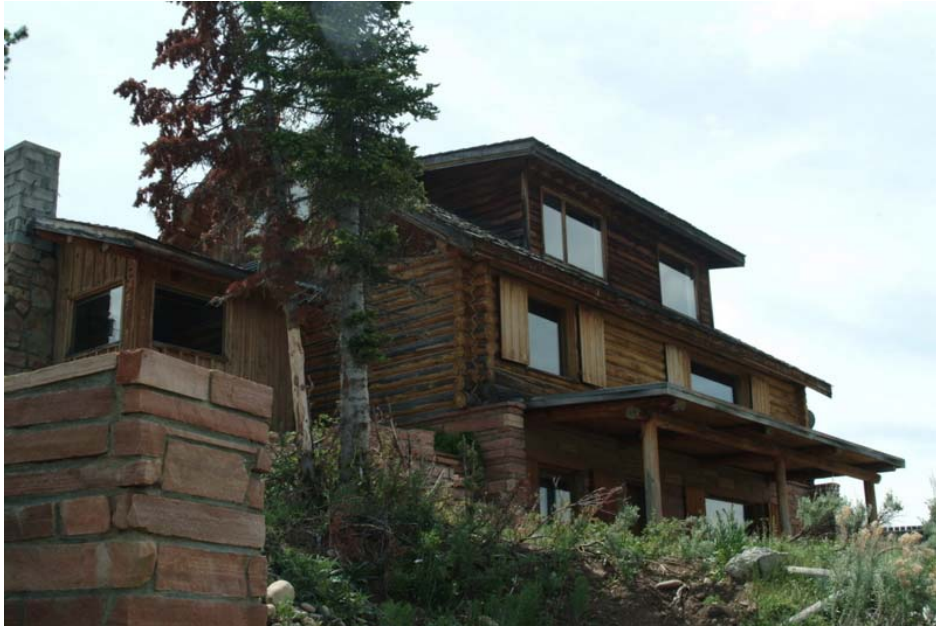
Rudd House, north and west elevations (Mary Humstone, 2007)
