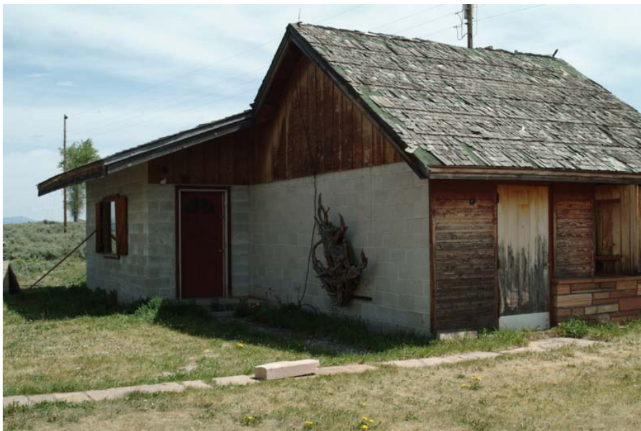
Rudd Garage/shop, south and west elevations (Mary Humstone, 2007)
