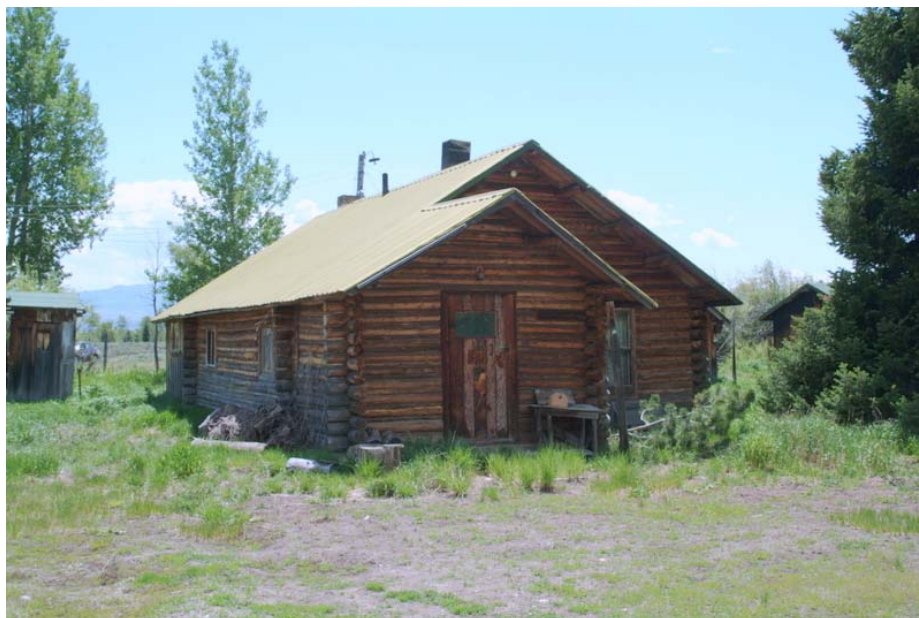
Hartgrave Cabin (Bldg. #6), west and south elevations (Mary Humstone, 2007)
