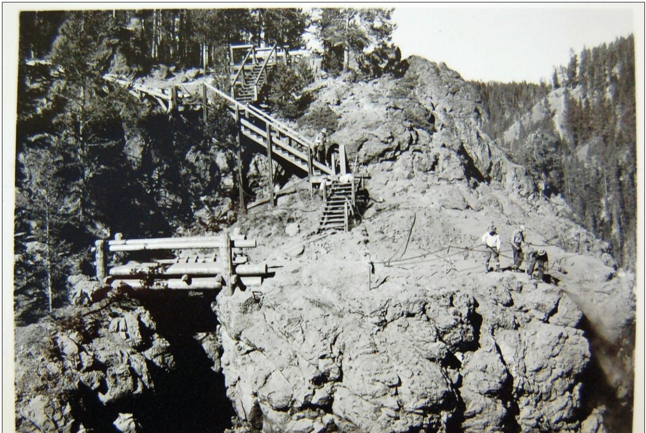
Brink of Upper Falls Overlook. "Trail bridge constructed and preparing site for parapet and platform." (Source: Final Report Reconstruction of Observation Platform – Canyon, Project FF 601 , by C.A. Lord, Park Engineer, 1937. Box K-30, File D66, Heritage Research Center, Yellowstone National Park)
