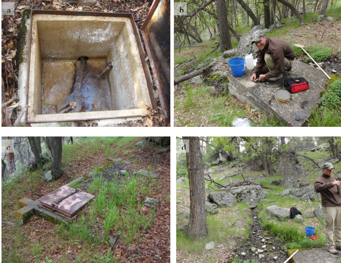
Figure 6. Waterline Spring consisted of 3 boxes and a stream: a.) Box 1, the upper most box, was a junction box where 2 pipes came together, b.) Box 2 contained little water, c.) Box 3, the lower box, was a large box full of water, and d.) a spring stream originated under a rock near Box 1.
