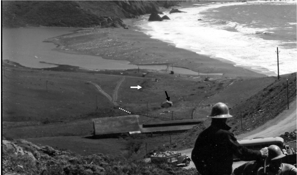
Figure 3. March 25, 1938 oblique ground photo looking south, showing the transverse road crossing (white dotted line) and a building (black arrow) next to a willow-lined channel. The channel extends beyond the building towards the ocean as seen prominently in figure 2. The white arrow highlights a channel in what appears to be the topographic low and natural historic main drainage area.
