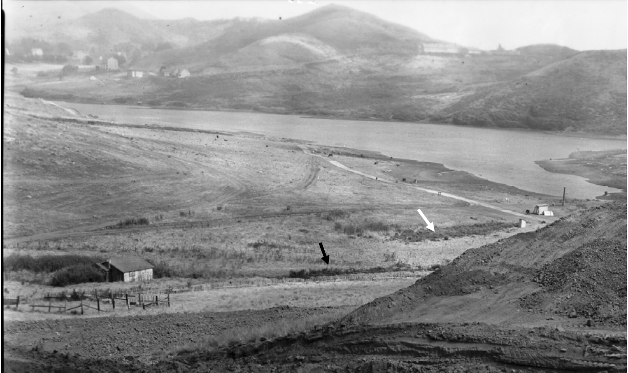
Figure 4. August 31, 1938. Looking southeast to the area down valley (south) of the ranch road (out of frame left). Arrows highlight drainage features visible in Figures 2 and 3. Black arrow shows a ditch below the small building. White arrow points to a natural historic drainage.
