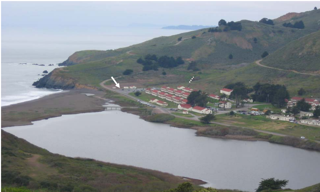
Figure 1. 1913 photo (top) of the Rodeo Beach wetland complex and ranch buildings, matched in March 2007 (bottom). White arrows indicate the location of the Surfer parking lot, which appears to have been a wet meadow in 1913. White dotted lines indicate the transverse ranch road location.
