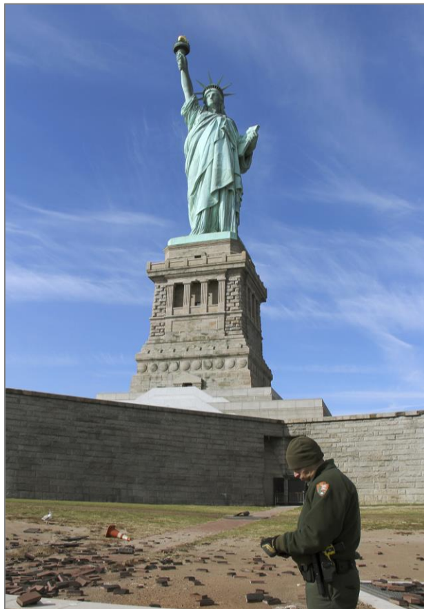
Photo 3. A National Park Service ranger surveys damage from the aftermath of Hurricane Sandy at Statue of Liberty National Monument, NY. Photo credit: National Park Service.
